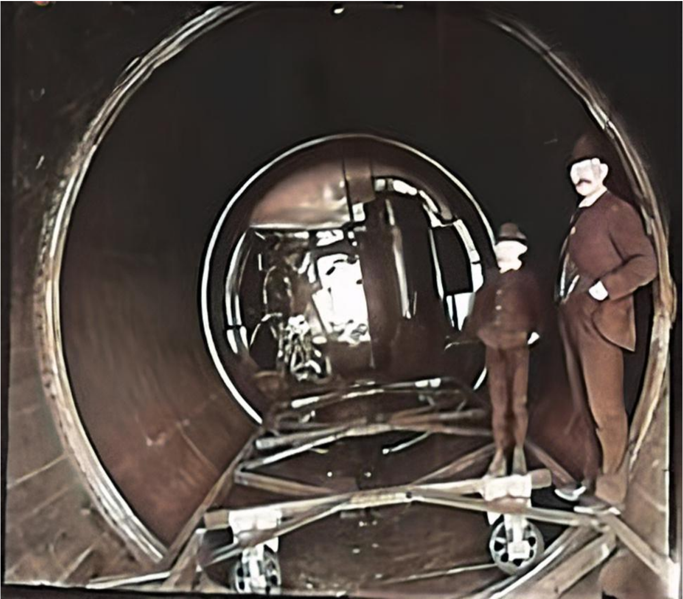
Inside the Roller Boat: The steam engine and boiler are clearly visible at the back. The unit is very small, given the work required, a Polson product, around 10-14 hp. The man is possibly John B. Miller and son Henry, who would have been 10 at the time.
