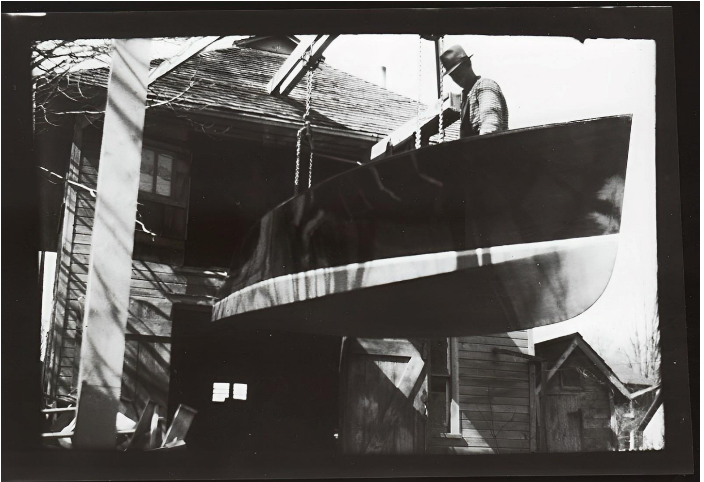
The boats were built in the second story and lowered onto a trailer when complete. Photo Manotick Classic Boat Club Archives
