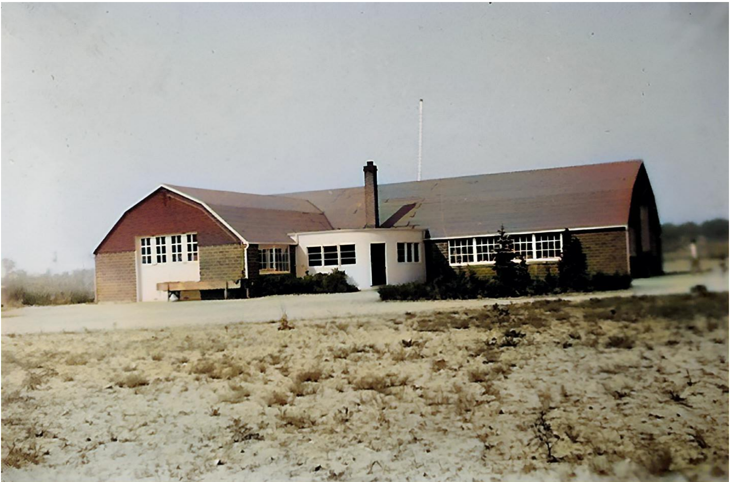
The new plant at Niagara on the Lake, the production line wing at the left with the garage doors, the finishing wing on the right with the four windows, the administration office in the semi-circular structure.
