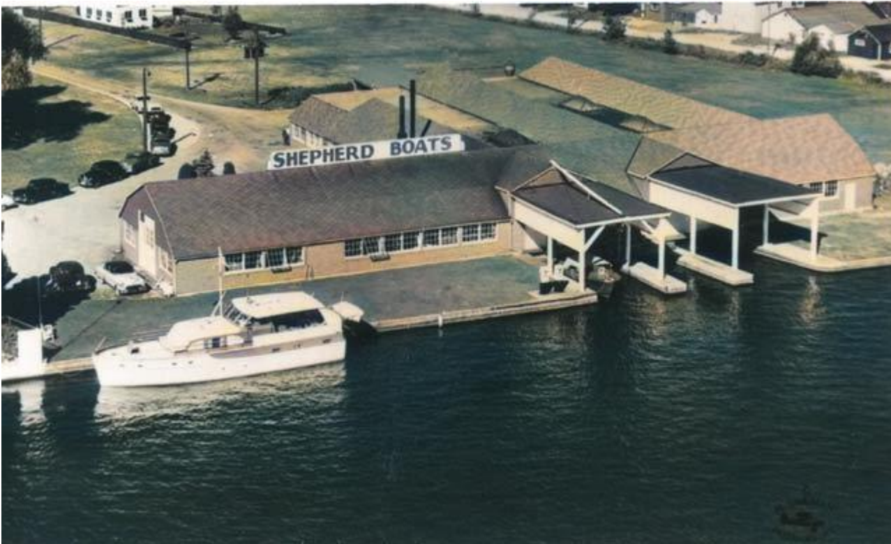
The final version of the works, Circa 1955, with a second production line, expanded finishing room (under sign) and showroom at top left of photo.
