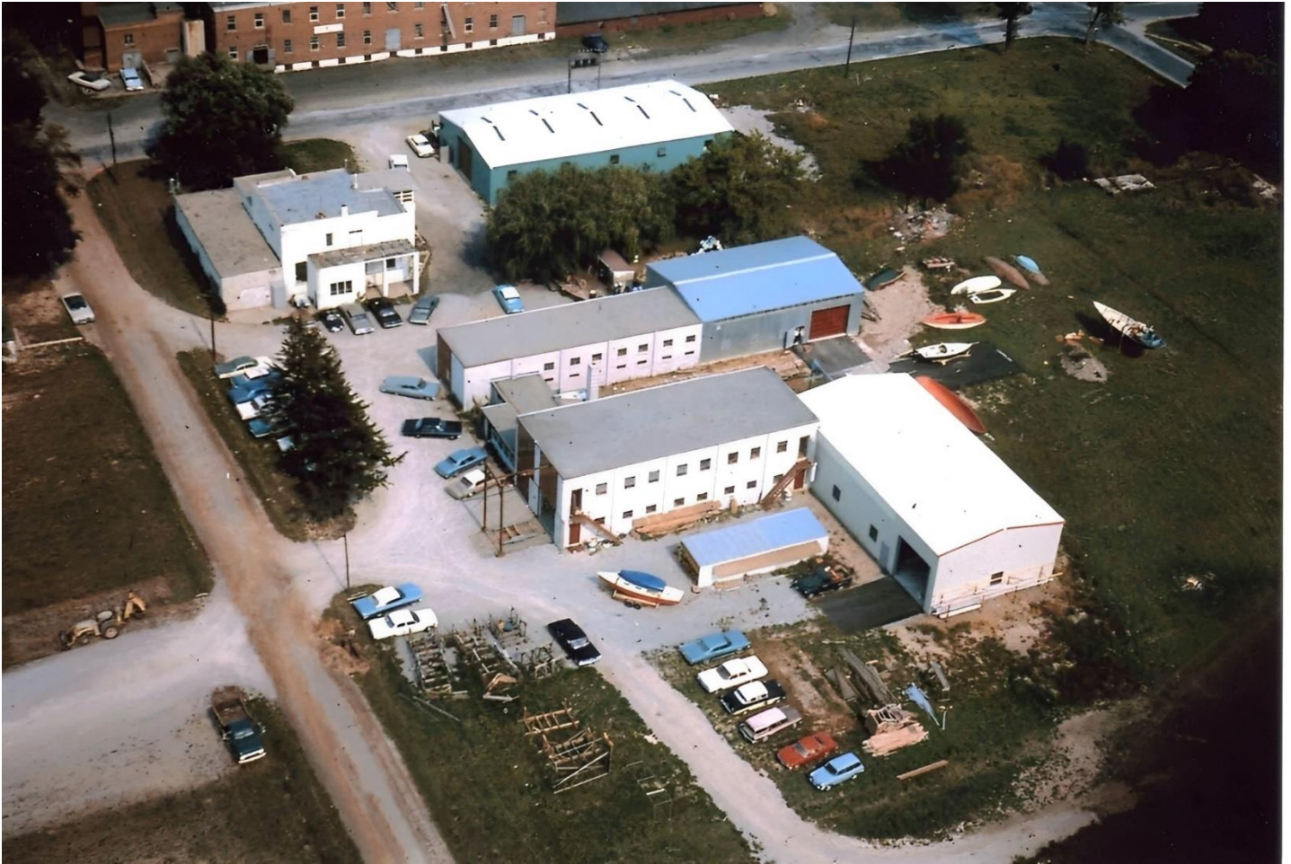
The main C & C plant complex at 526 Regent Street, Niagara on the Lake, 1979 Photo niagaranow.com
