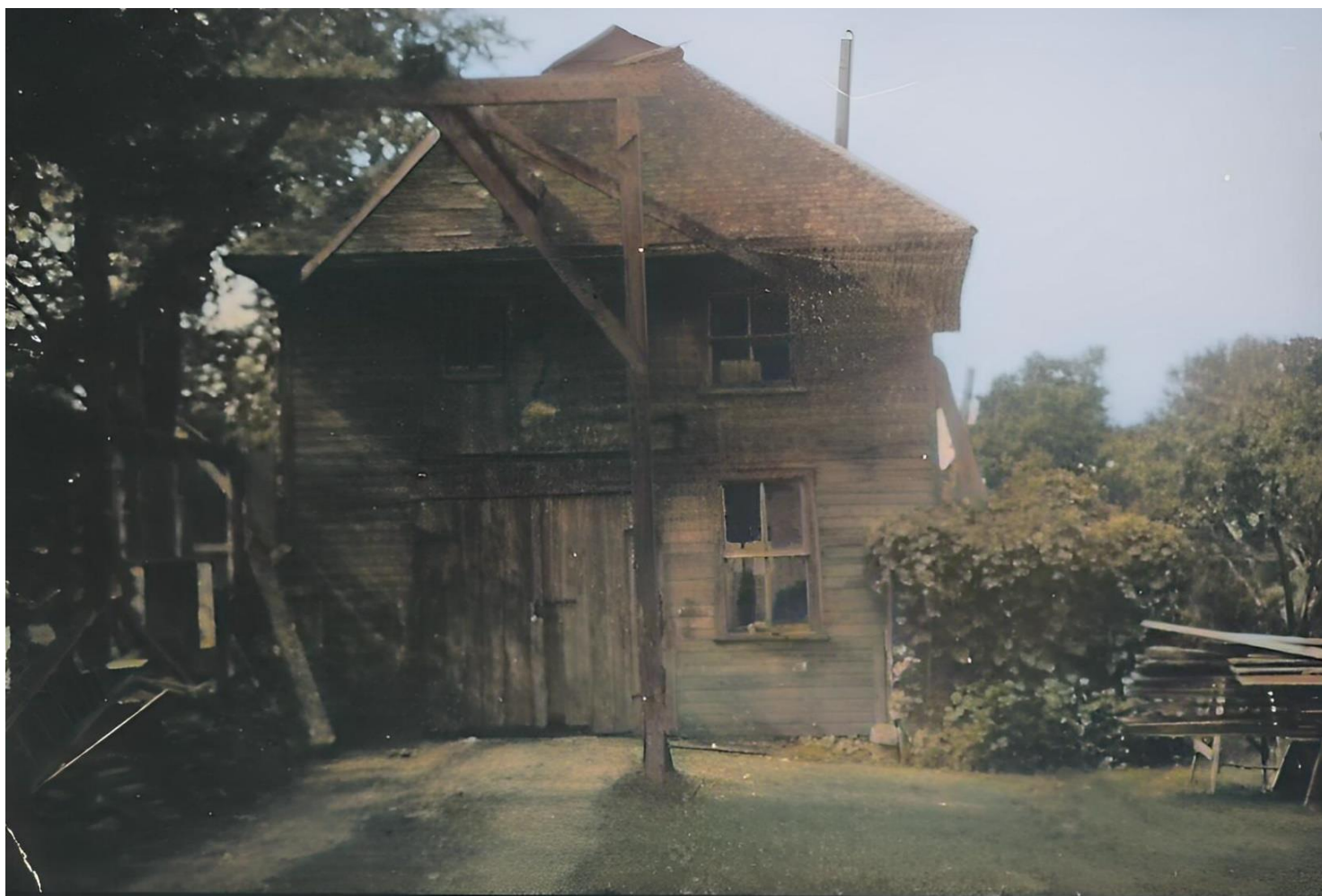
Jeffrey's Athens workshop, with boat hoist in place
